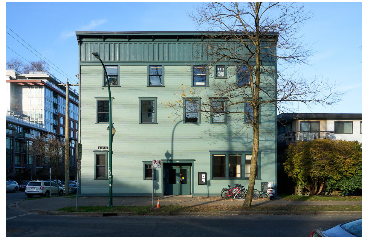
Western Front, 303 E 8th Ave, Vancouver, 2026
